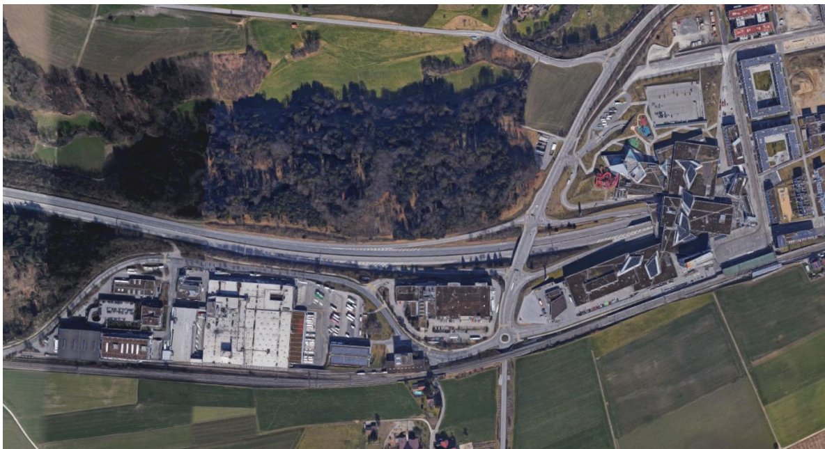
Illustration 10: Centre commercial et de loisirs Westside, Berne (Source: Google Maps)
